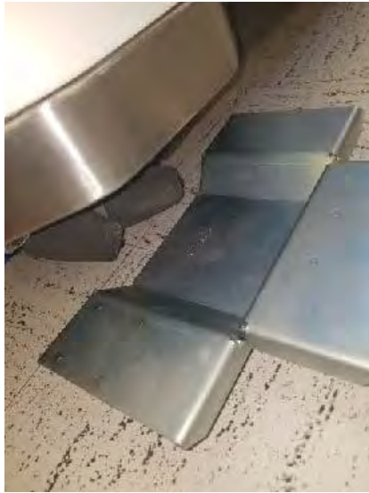
Figure 294: Move the dollies into place
