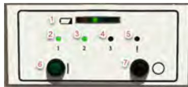
Figure 410: SDS control panel and description of components
